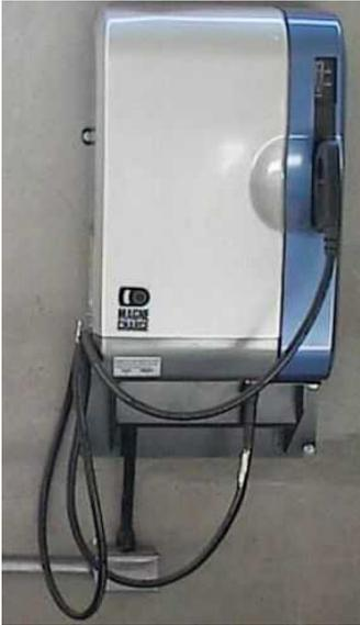
The photo in Figure 2 is of the TAL 2000 Small Paddle Inductive charger, included with each RAV4-EV. These are 208/240 VAC powered units, and require the equivalent of an electric dry connection in residential installations.
